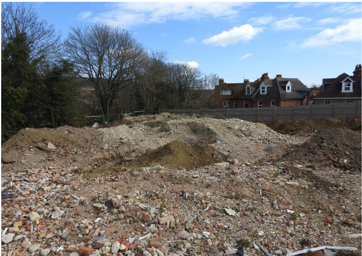
Plate 2: Showing north-eastern part of the site. Looking north-east.
