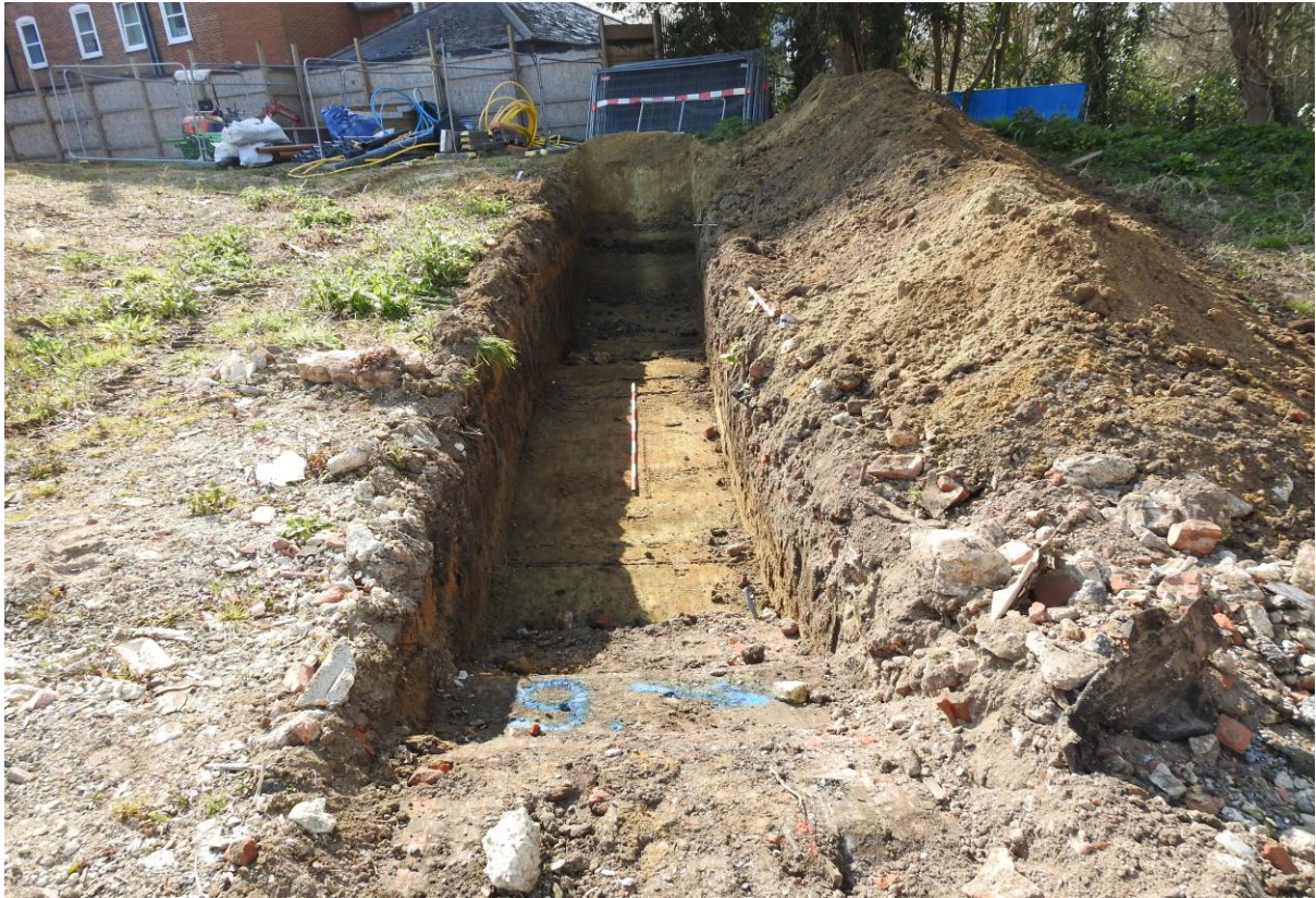
Plate 15: Showing evaluation Trench 9. Looking west with two-metre scale.
