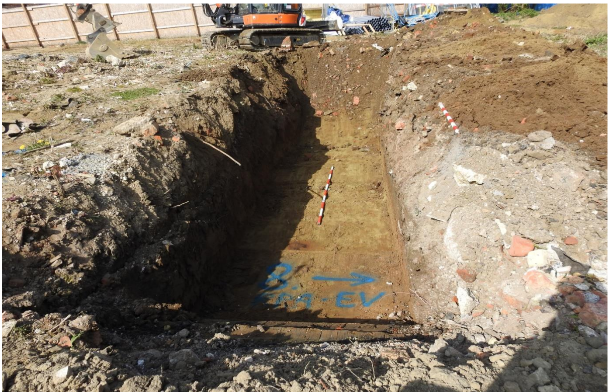
Plate 14: Showing evaluation Trench 8. Looking west with two-metre scale.
