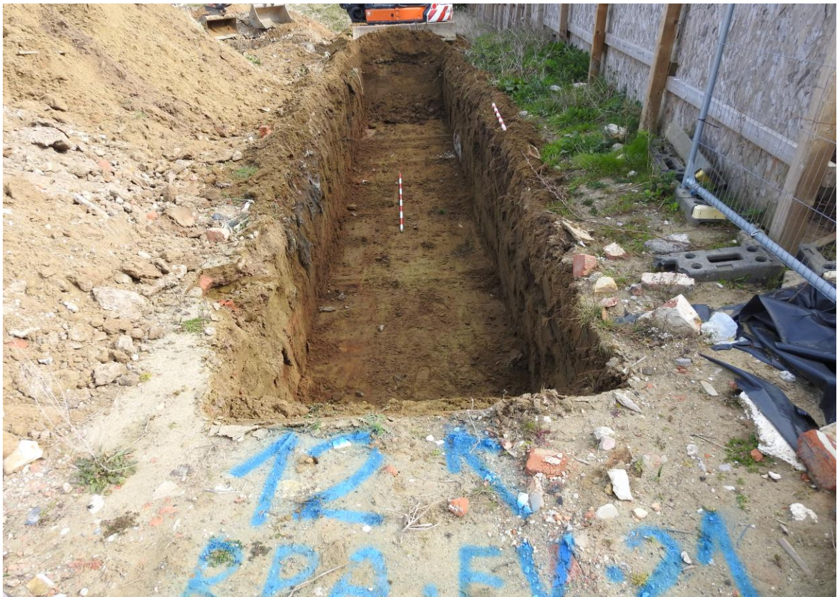
Plate 18: Showing evaluation Trench 12. Looking north-east with two-metre scale.
